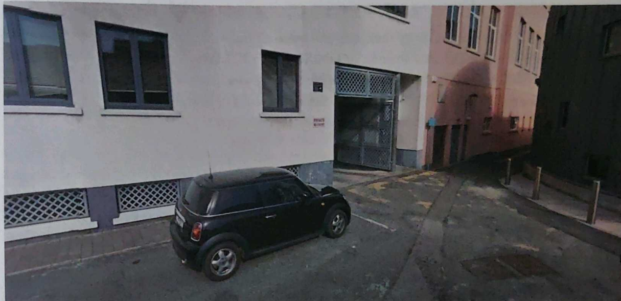
Figure 6: Entrance to Government Offices at Nunn's Lane
